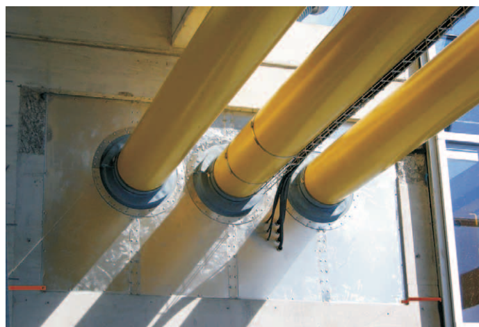
Fig. 19: Wall sealing
